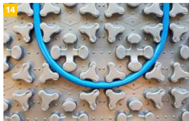
14 The heating cables are routed around the crossbones, which protects them.
