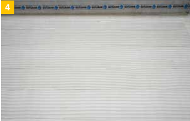
4 Apply adhesive using a suitable trowel notch.
