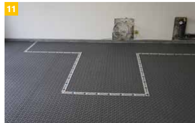
11 Heat-free zones must be marked before laying the heating cables and left clear. These must be marked on the enclosed laying plan (see laying plan).
