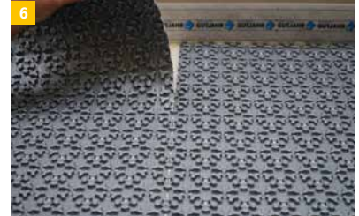
6 Fit together with a butt joint.
