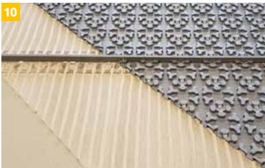
10 The support mats must be separated at structural separation and expansion joints. The formation of joints must take place in accordance with the regulations and manufacturer specifications of the appropriate fluid floor filling compound and the floor covering.
