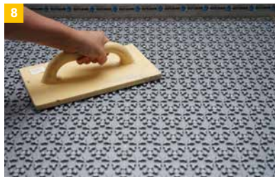
8 Press on or roll on the IndorTec® THERM-E over its entire surface.
