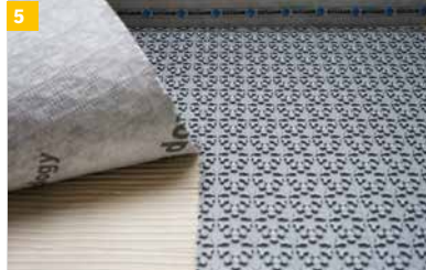
5 Embed the IndorTec® THERM-E which has been cut to size in the adhesive together with the fleece.
